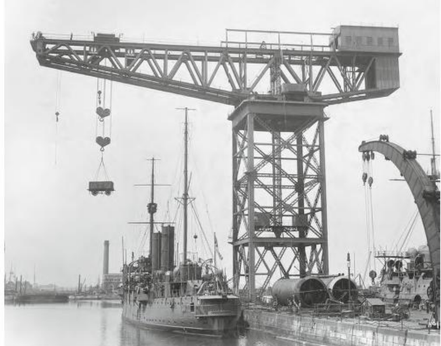
Plate 14: Giant Cantilever Crane, HM Dockyard, Portsmouth, England [N23]. General view of completed crane, 1912 (NMRS Image No. SC355126).
