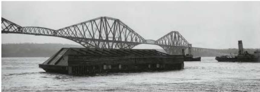
Plate 10: Rosyth Dockyard. Tugs taking charge after the launch of one of the seven sliding dock caissons designed and built by Arrol for the Admiralty, en route from the construction site at North Queensferry to Rosyth Dockyard, c. 1914. In the background, the Forth Railway Bridge, Sir William Arrol and Company's most famous project (1882-1890).
