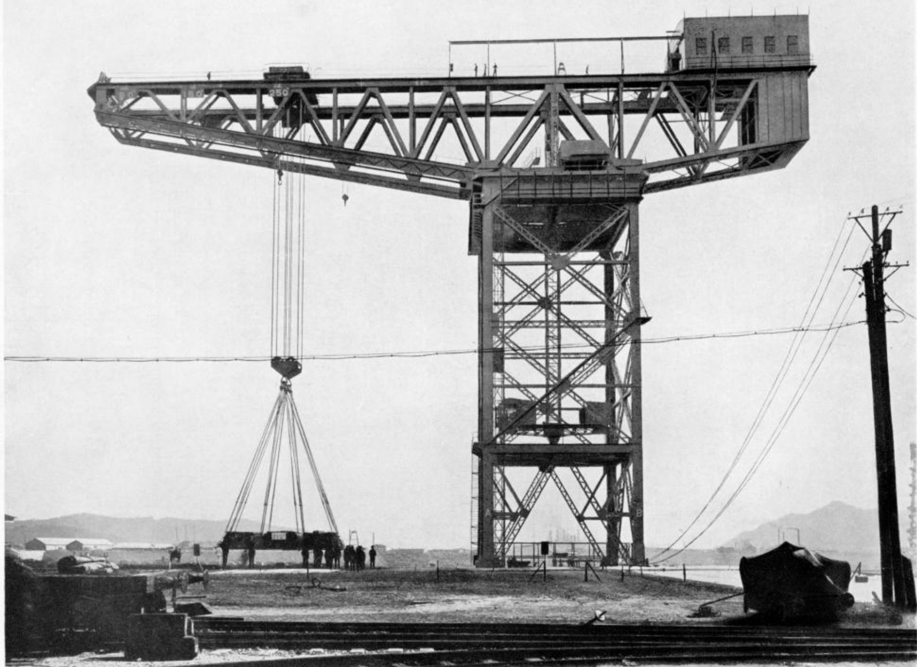
250-ton Giant Cantilever Crane, with Slewing Motion.
