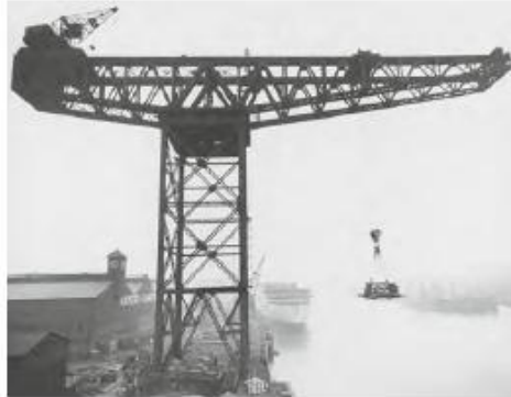
Plate 9: Giant Cantilever Crane, Walker Shipyard, Newcastle-upon-Tyne, England [N21]. View of crane undergoing testing with 250-ton load, 1931 (NMRS Image No. SC355113).
