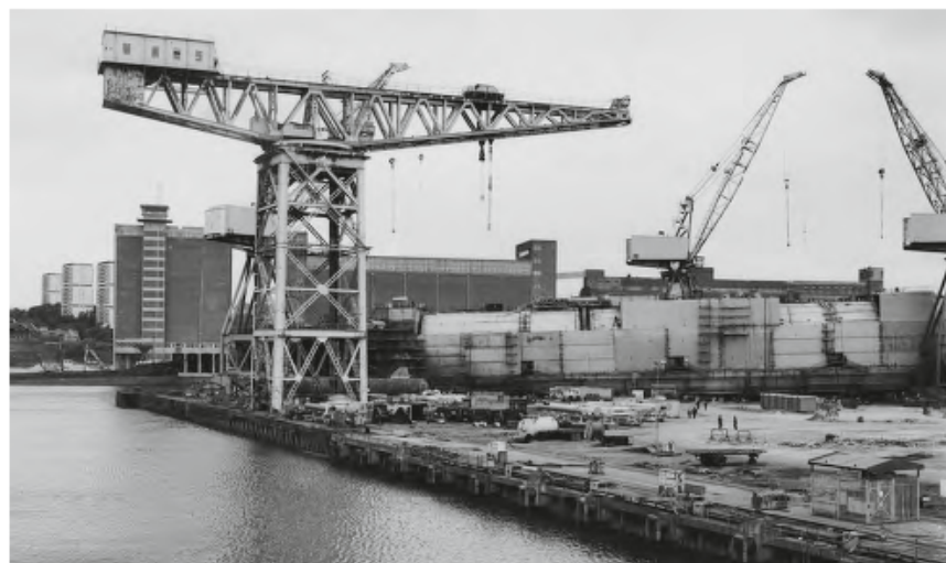
Plate 18: View from south-south-west across the fitting-out basin of the former Fairfield Shipyard in Glasgow (now Kvaerner Govan), showing the Arrol 220-ton Giant Cantilever crane (built in 1911) (B 41310, 1990, RCAHMS, item 74).
