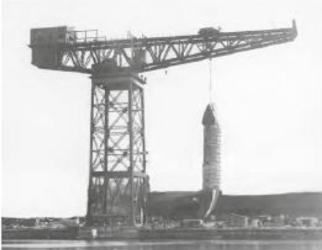
Plate 8: 150-ton Giant Cantilever Crane, Barrow-in-Furness, England [N18]. General view lifting test load of 182.5 tons at maximum radius of 85 feet, 1942. This replaced an earlier crane built by the Glasgow Electric Crane and Hoist Co. which was destroyed in an air raid in May 1941. (NMRS Image No. SC355111).
