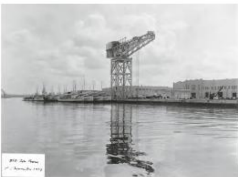
Plate 10: 250-ton Giant Cantilever Crane, Singapore Harbour [N12]. General view of crane on completion at Singapore, 1938 (NMRS Image No. SC355107).
