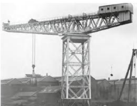
Plate 12: Giant Cantilever Crane, North East Marine Shipyard, Wallsend, England [N22]. View of completed crane with test load of 187 tons, 1909 (NMRS Image No. SC355120).
