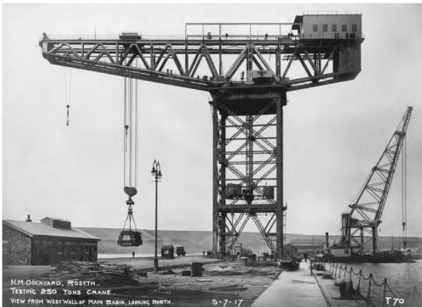
Plate 11: 'HM Dockyard, Rosyth Testing 250 Tons Crane... 5.7.17'. The acquisition of the Porthead Crane Works in 1910 allowed Arrol not only to design and build such cranes, but also to provide the machinery (C 87838 PO, item 32).
