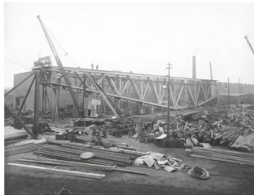
Plate 61: 250-ton Giant Cantilever Crane for the Japanese Imperial Dockyard, Sasebo [N11]. View of the crane jib assembled outside Arrol's Parkhead Works, Righy Street, Glasgow in 1912. The Japanese clients can be seen inspecting the work on top of the jib (MARS Image No. SC555100). See also Figure 2.
